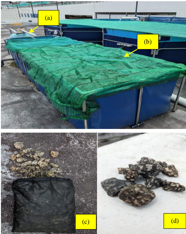
Fig. 2. Components in filtration section: (a) sand filter, (b) biofilter tank, (c) agrogeology rocks in mesh bag, and (d) agrogeology rocks.
